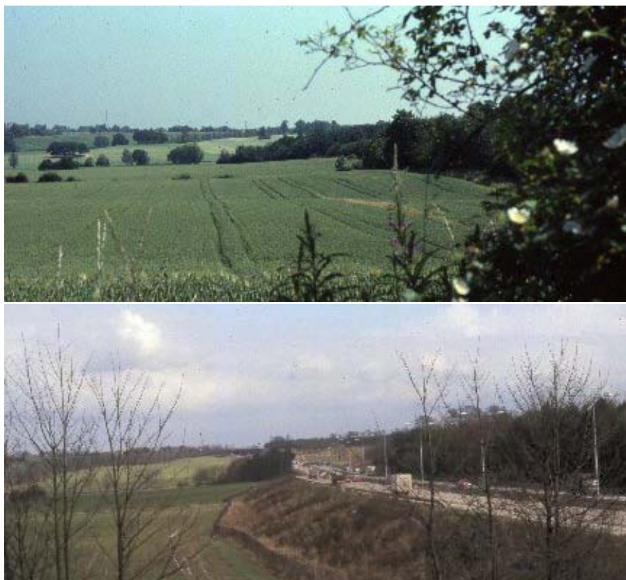
Route of the M25, looking towards the Epping tunnel from the Copped Hall Track - before & after construction
