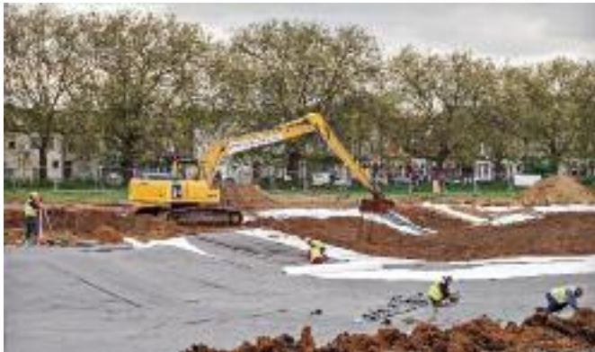
Jubilee Pond as it appeared several months ago, when a new liner was put in place. Photo: Bob and Sandy Gibbons
