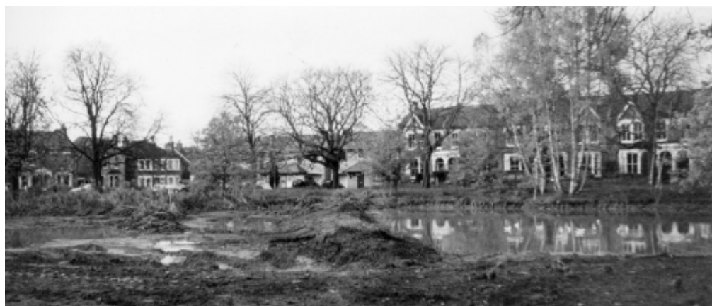
St John's Pond during silt removal
