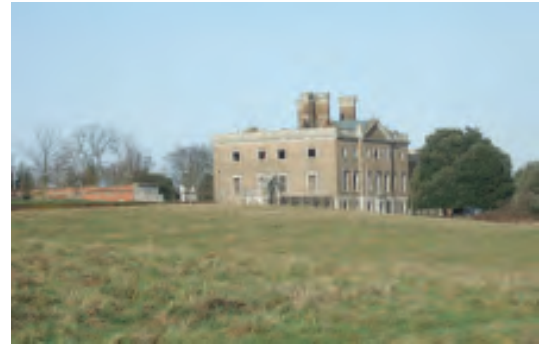
View of Copped Hall from below the ha ha
